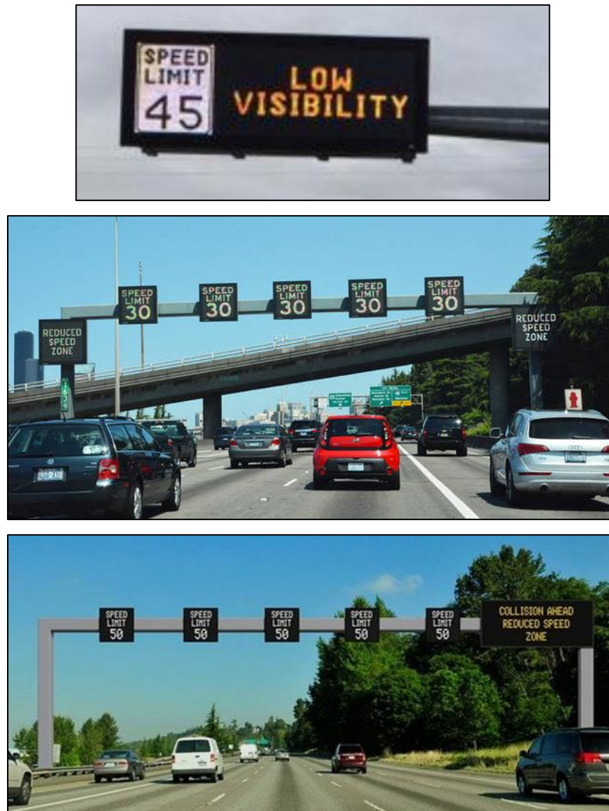
Figure 4.6: Example Overhead Gantries with Variable Speed Limit and Dynamic Message Signs
