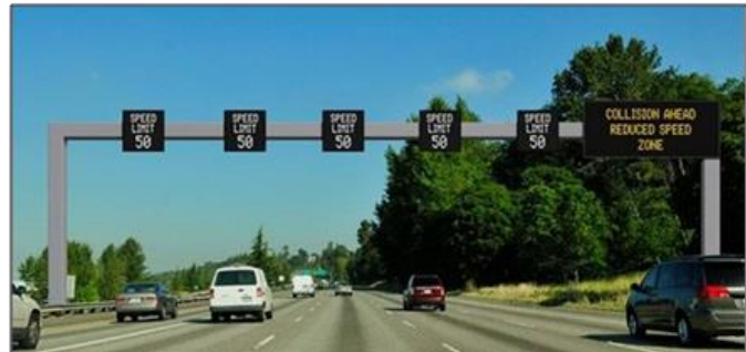
Figure 4.11: Example of Queue Warning DMS
