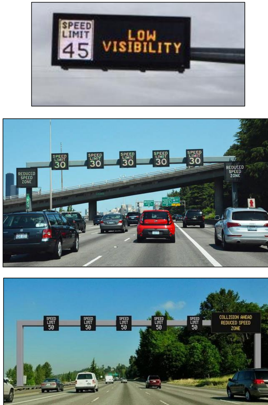
Figure 25: VSL and Small DMS Sign Examples
