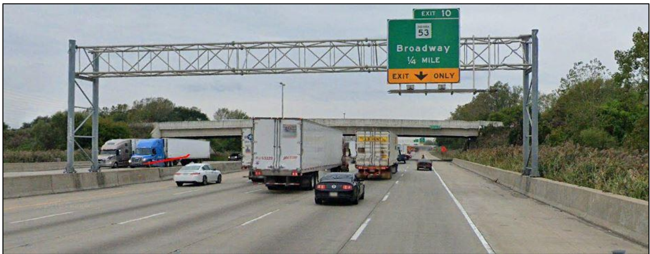
Figure 20: Existing Sign Truss at Exit 10/Broadway
