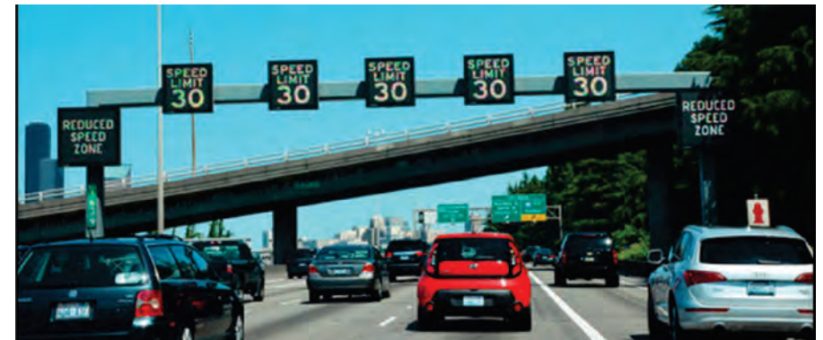
Variable Speed Limits and Queue Warning
