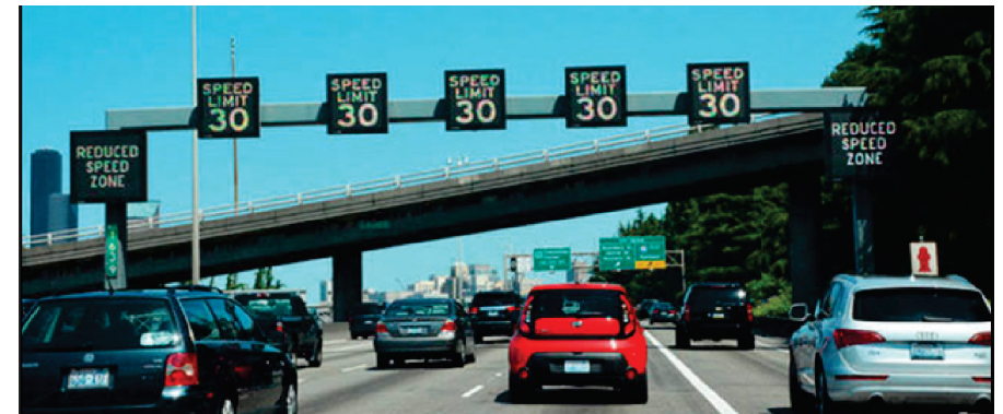
Variable Speed Limits and Queue Warning
