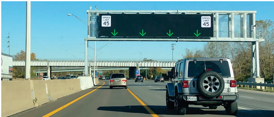
A combination of lane control, hard shoulder running, and variable speed limits
