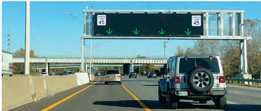
A combination of lane control, hard shoulder running, and variable speed limits
